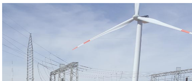
Fig.7 Wnd substation and Wind Turbine
